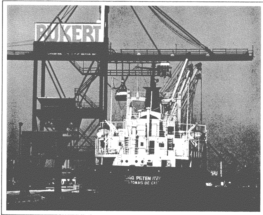
Considered as the most sophisticated in the industry, the Rukert bulk cargo crane can travel 450 feet up and down Pier 5.
