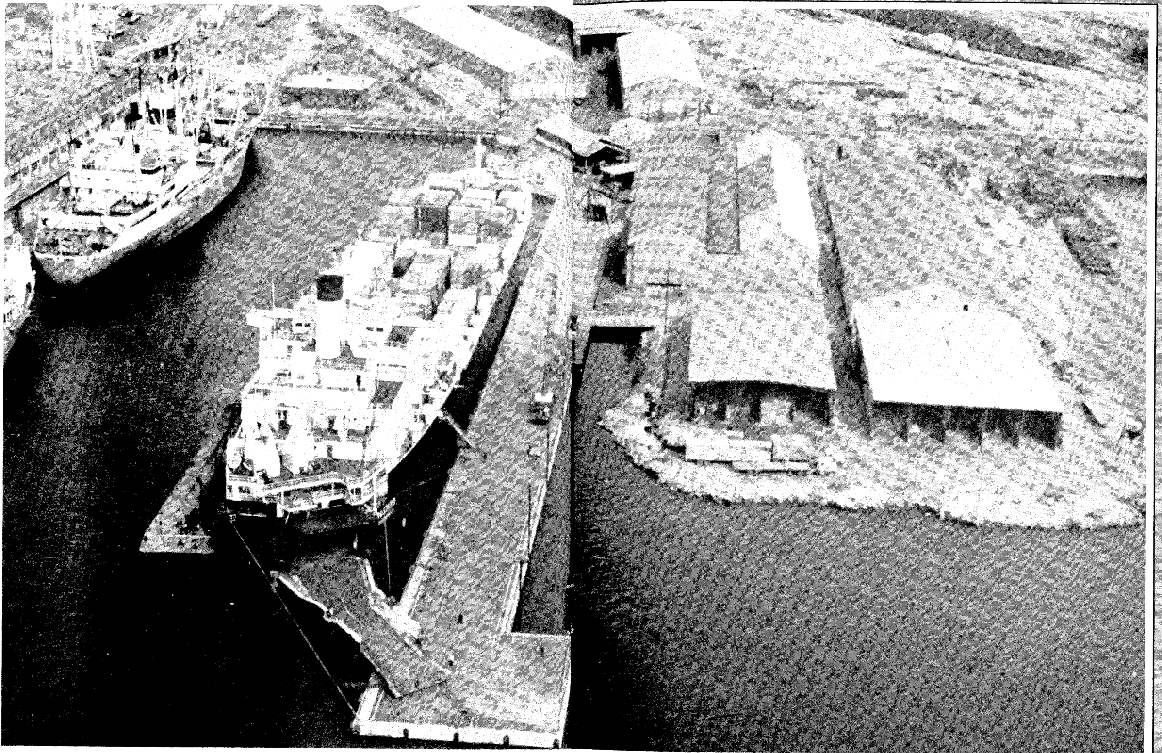
The Pier 5 terminal as completed in 1981.
