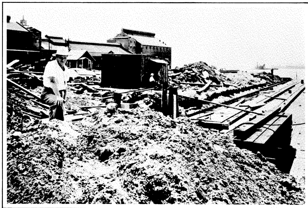
The first major post-war construction, building "A" berth Lazaretto in 1953.
