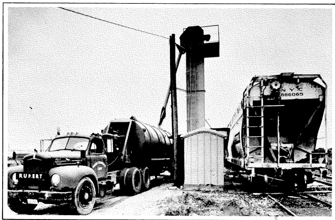
Bulk phosphates for Baltimore soap plants are transferred from rail sidings into trucks in the late 1950's.
